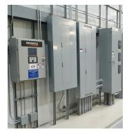
An Automatic Transfer Switch is used for switching power between the utility and the generator. The automatic transfer switch will monitor incoming voltage from the utility, and if there is an interruption, the transfer switch immediately senses the problem and signals the generator to start. As the generator begins to run, the automatic transfer switch safely shuts off the utility feed and at the same time opens the generator power feed.
