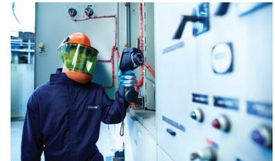
Ultrasonic testing is an excellent tool for flaw detection, such as finding compromised wiring within conduit. Using ultrasonic technology to detect and correctly identify these electrical anomalies can help prevent electrical failures and reduce life and safety risks. Ultrasonic is especially effective when used in conjunction with infrared thermography to deliver a thorough condition of maintenance assessment.
